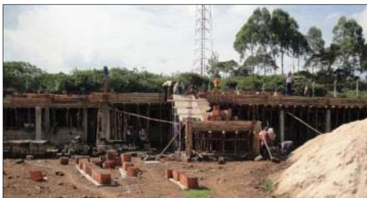
New Primary School under construction, BBCEC
